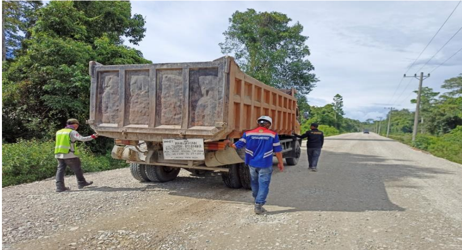
Gambar 3. Proses uji test proof rolling
